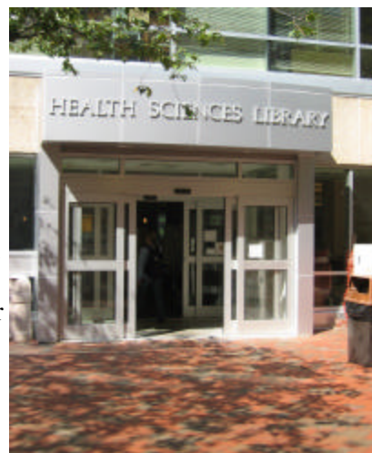
The renovated entrance facing MacNider features a brushed metal facade, new windows, and brick paving.
